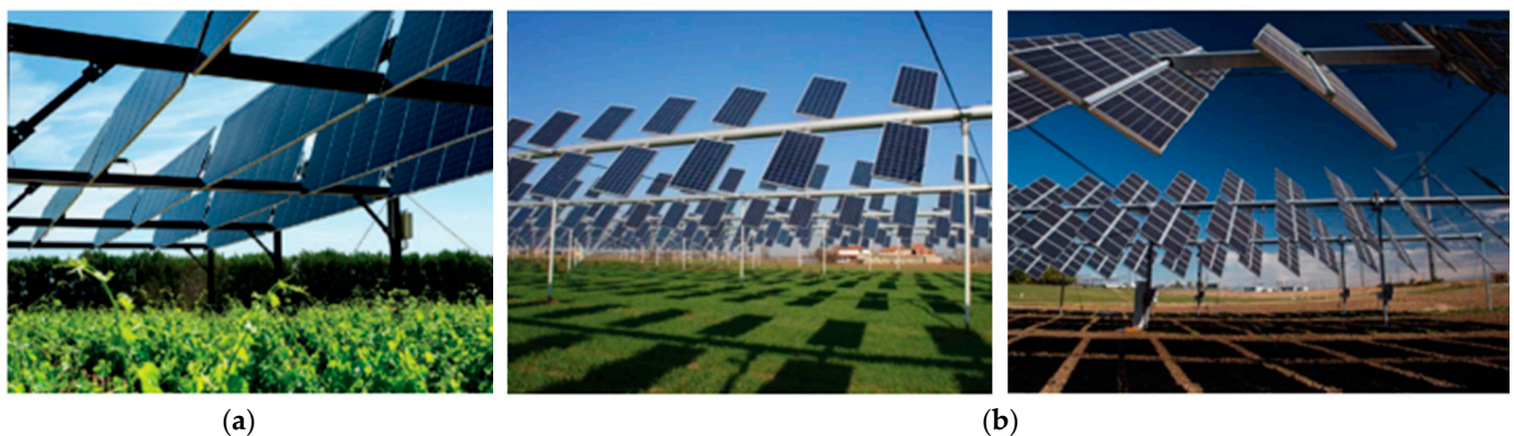
Figure 7. (a) Single-axis solar tracker module [44] and (b) dual-axis solar tracker module [60].
